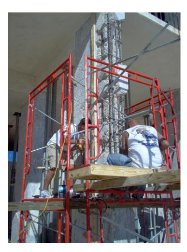
After cleaning of rusted steel a inorganic zinc coating is applied to all rebar, field applied galvanizing
