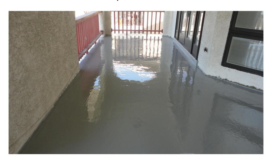
Applying Top coat of Vulkum waterproof membrane over repaired concrete with sand broadcast for non slip surface
